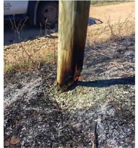
**Burning a pole could result in a widespread power outage and be costly for those responsible for the fire. The cost to replace just one utility pole can range from \$1,500 to \$2,500.**
