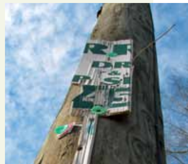
Staples, nails, and tacks used to hang signs pose dangers to Flint Hills RECA's linemen
